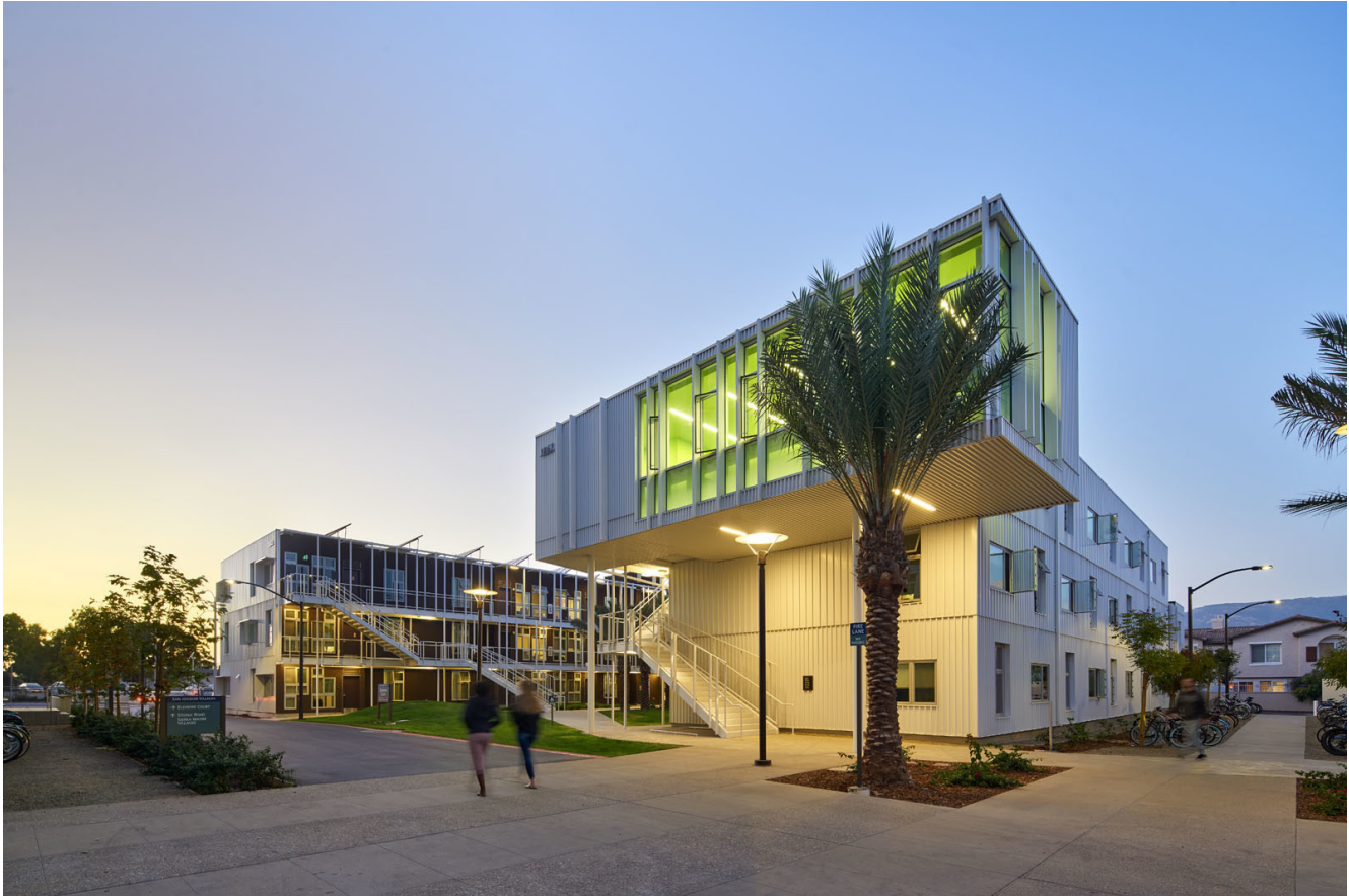
LOHA's dormitory for UC Santa Barbara, completed last year, staggers patterns and places stairways at angles, preventing the structures from feeling blocky. (Bruce Damonte / LOHA)
