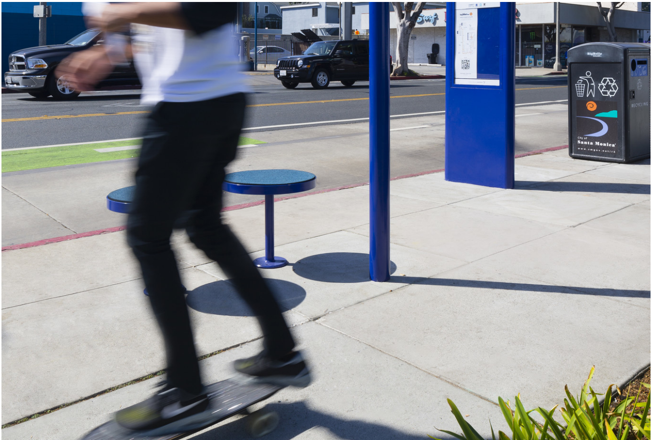
LOHA's design for the Big Blue Bus in Santa Monica in 2016 consists of shelters that can be sized according to need. (Lawrence Anderson / LOHA)
